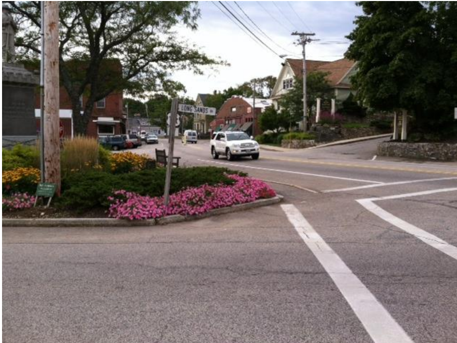
Signs Clutter Sight Distance View Looking Left
