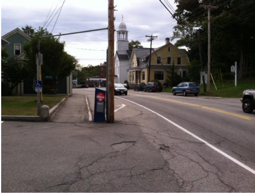
On-street Parking Restricts Sight Distance & Utility Pole Obstructs View
