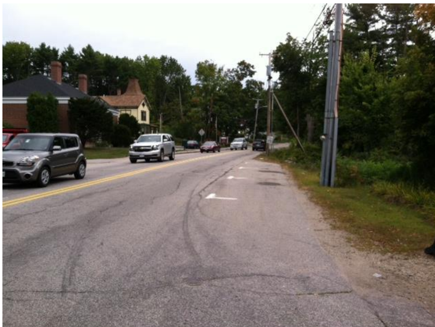
Looking North on Long Sands Road – Utility Poles
